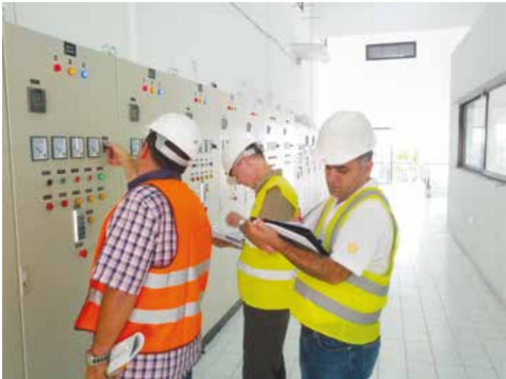
Panel Boards delivery, check and testing by client/consultant
