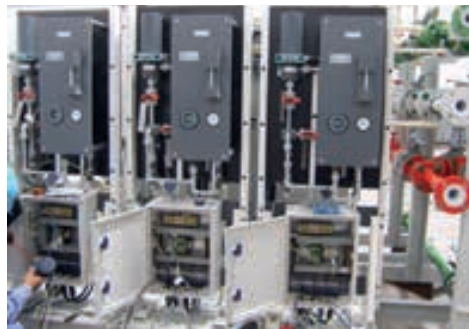
ABU DHABI, UAE (2007) Onshore gas development project Disinfection of fire water, service water and drinking water
