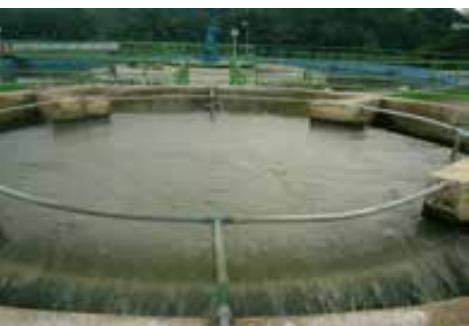
INDONESIA (2004) Municipal Water plant Water disinfection with gas chlorine
